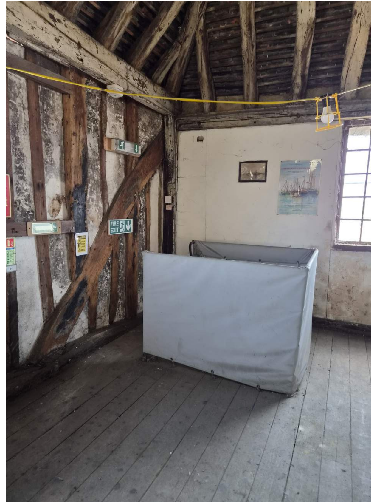
Figure 12. Existing ladder stair providing access between the ground and first floors, introduced during the building's twentieth century adaptation for Sea Cadet use.
