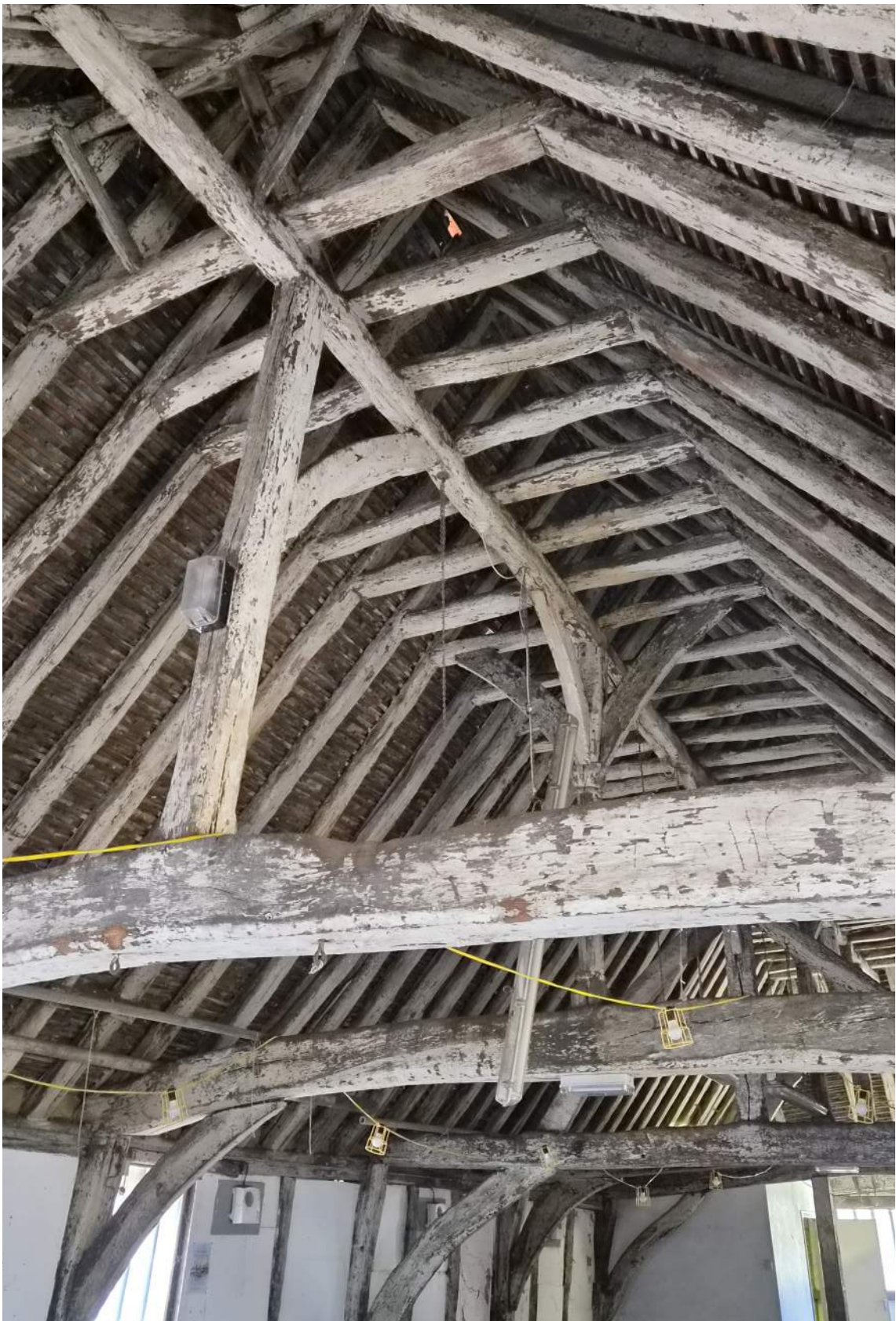
Figure 1. Existing timber roof structure viewed from the first floor.
