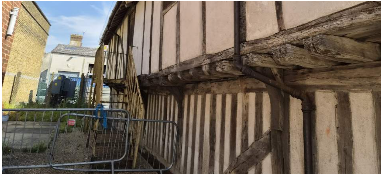
Figure 11. Existing metal staircase providing access to the first floor.
