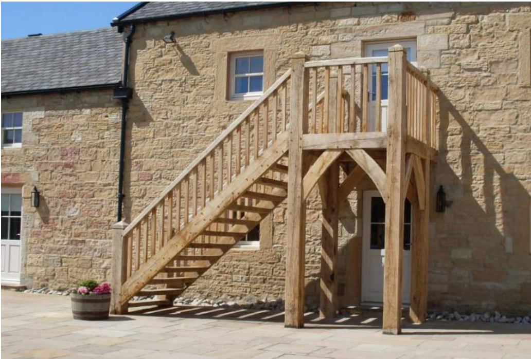
Figure 16. Precedent Study: External Oak Stair and Access Landing
