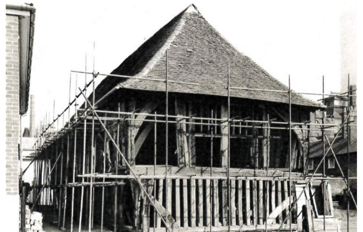
Figure 8. Repair and restoration works to the Old Town Warehouse in the early 1960s. Source: Anthony Swaine Architecture Ltd Collection.
