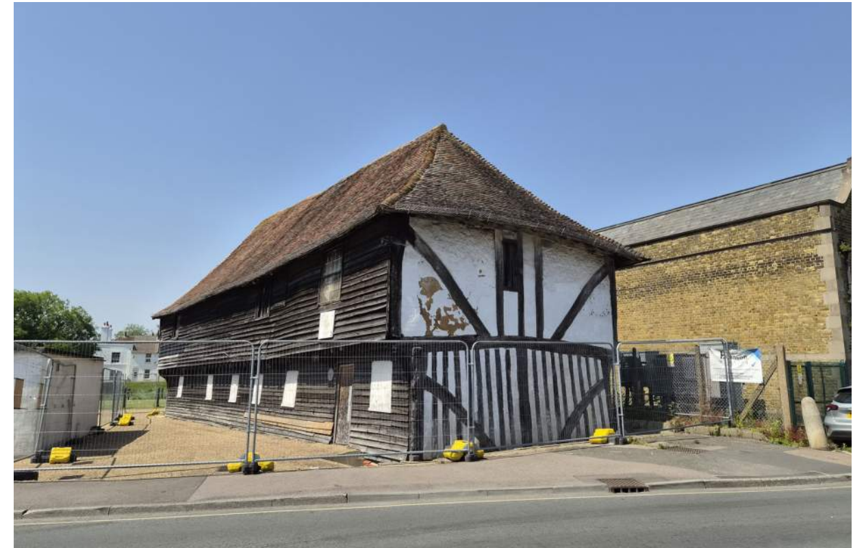
Figure 4. Existing building viewed from Conduit Street
