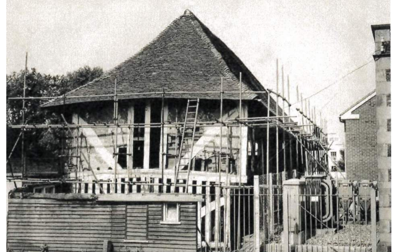
Figure 7. Repair and restoration works to the Old Town Warehouse in the early 1960s. Source: Anthony Swaine Architecture Ltd Collection.
