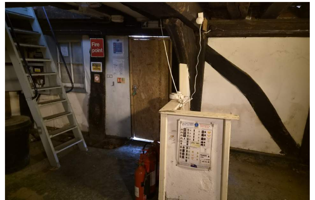
Figure 19. Recent opening up and investigation works to improve understanding of the building's construction.
