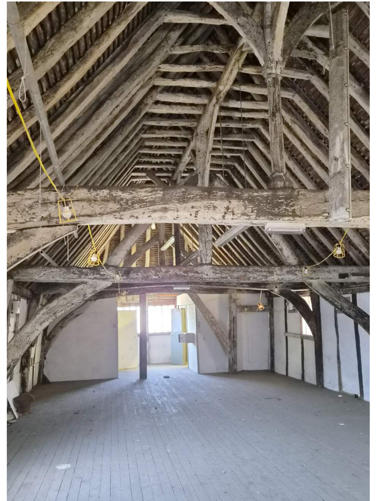
Figure 21. Existing interior of first floor.
