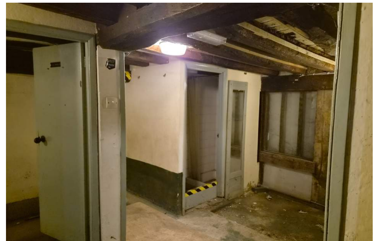
Figure 5. Existing building interior showing the entrance area and partitioning associated with the Sea Cadets' use of the building.
