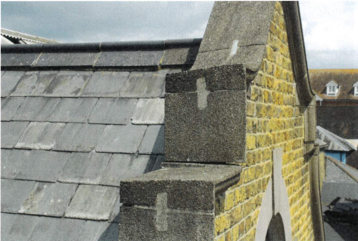
Structural movement to southeast gable.
