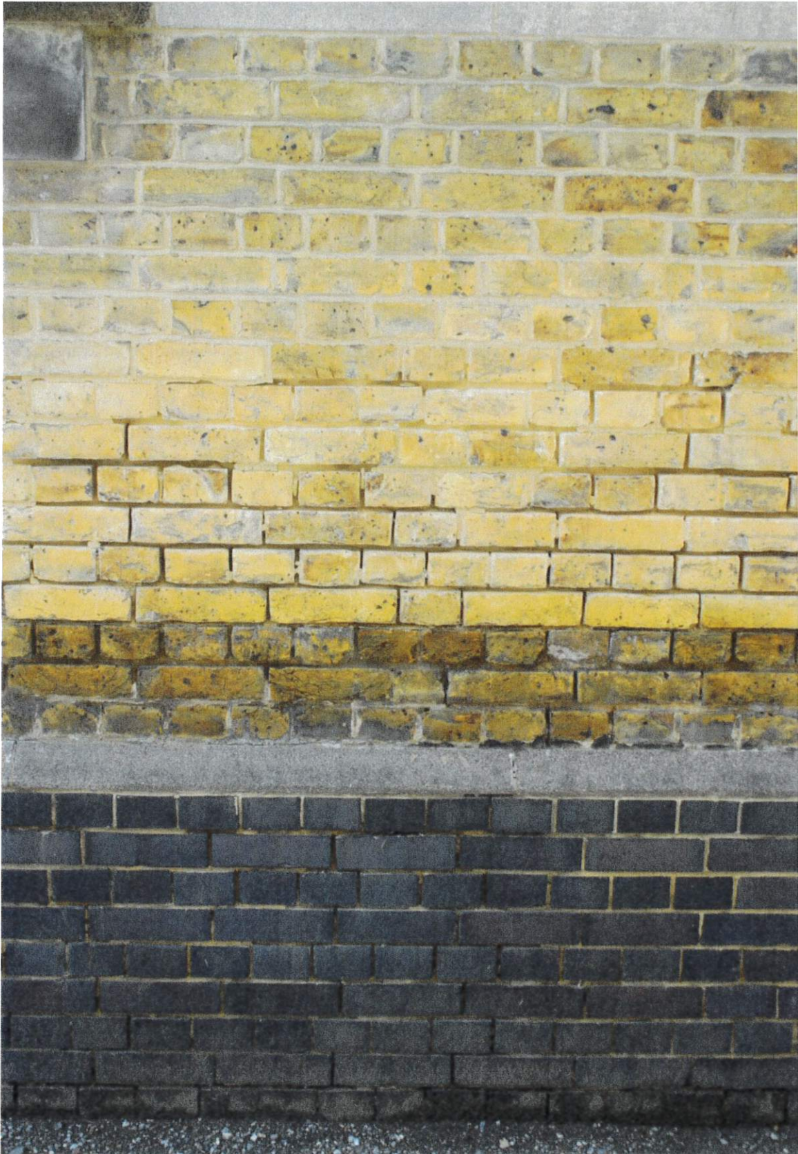
External wall construction.
