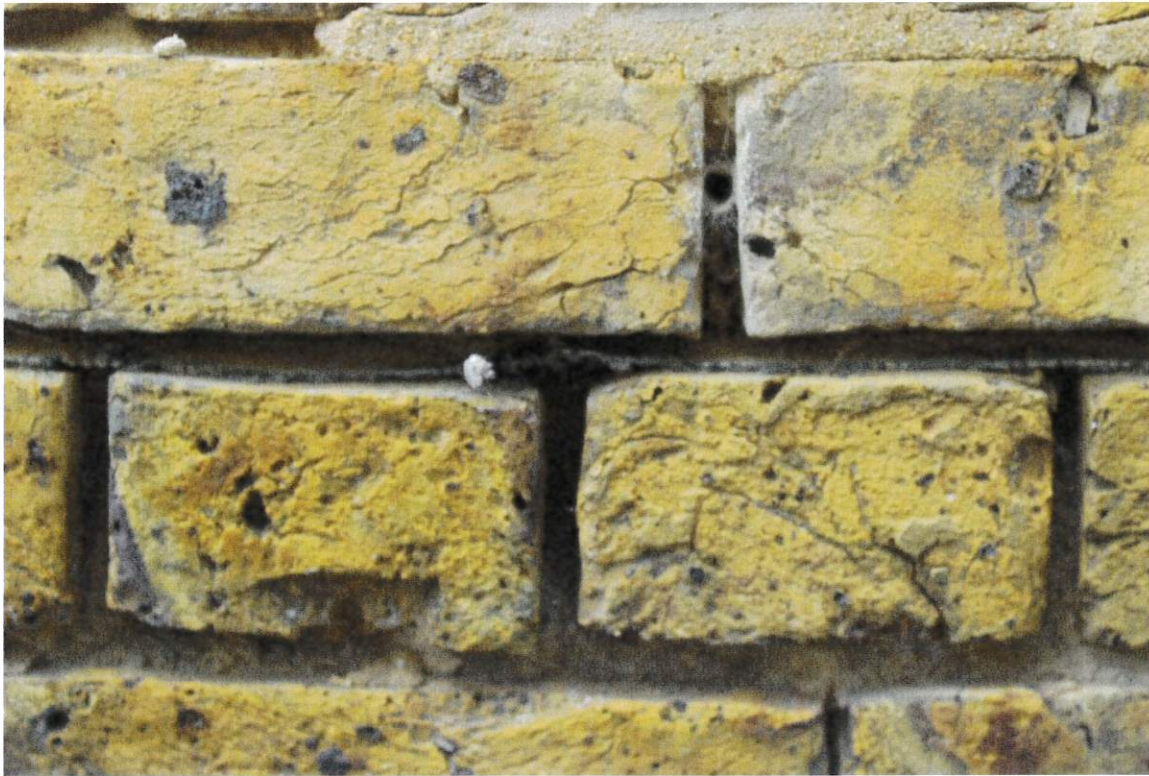
Bitumen DPC in flank walls. Is this linked to a DPM in the floor?
