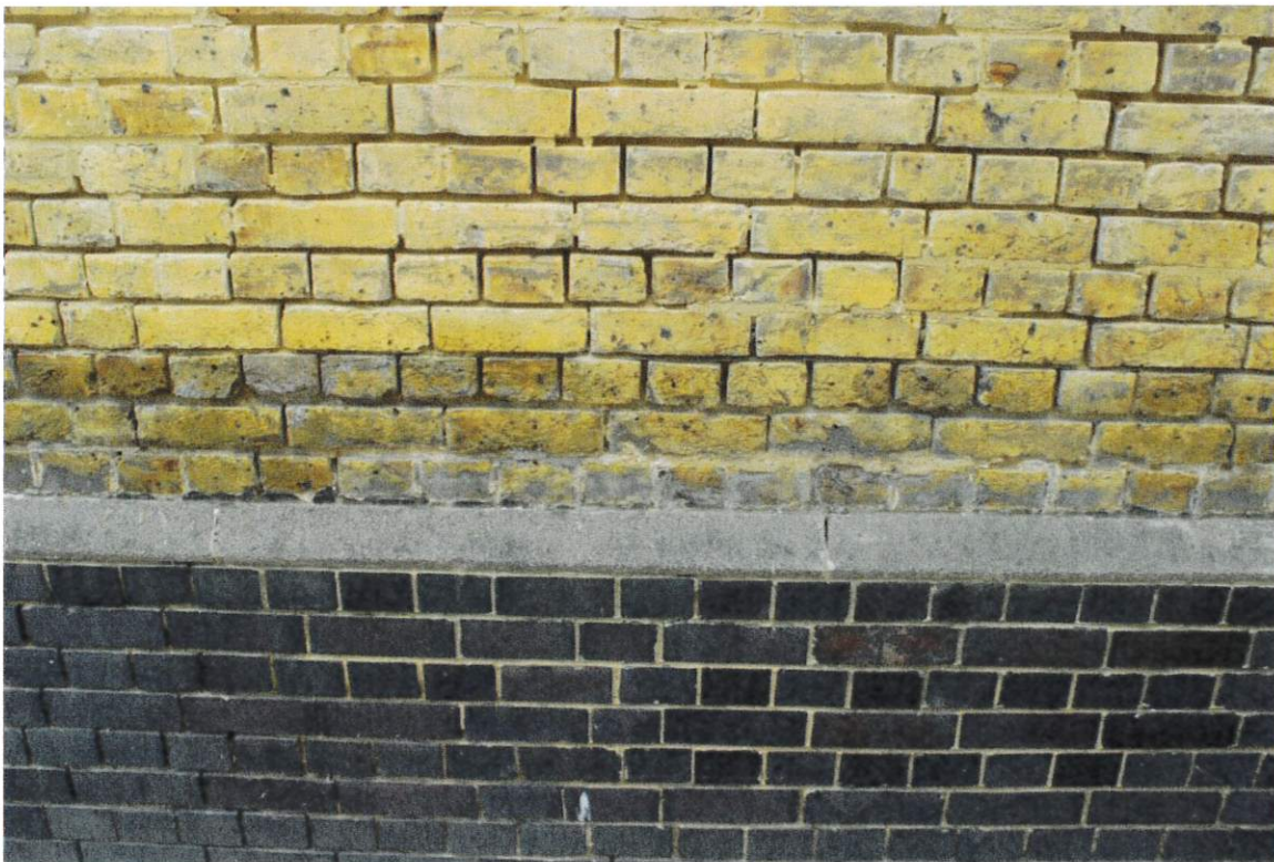
Bitumen DPC in flank walls. Is this linked to a DPM in the floor?
