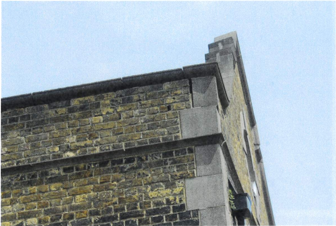
Structural movement to southeast gable.
