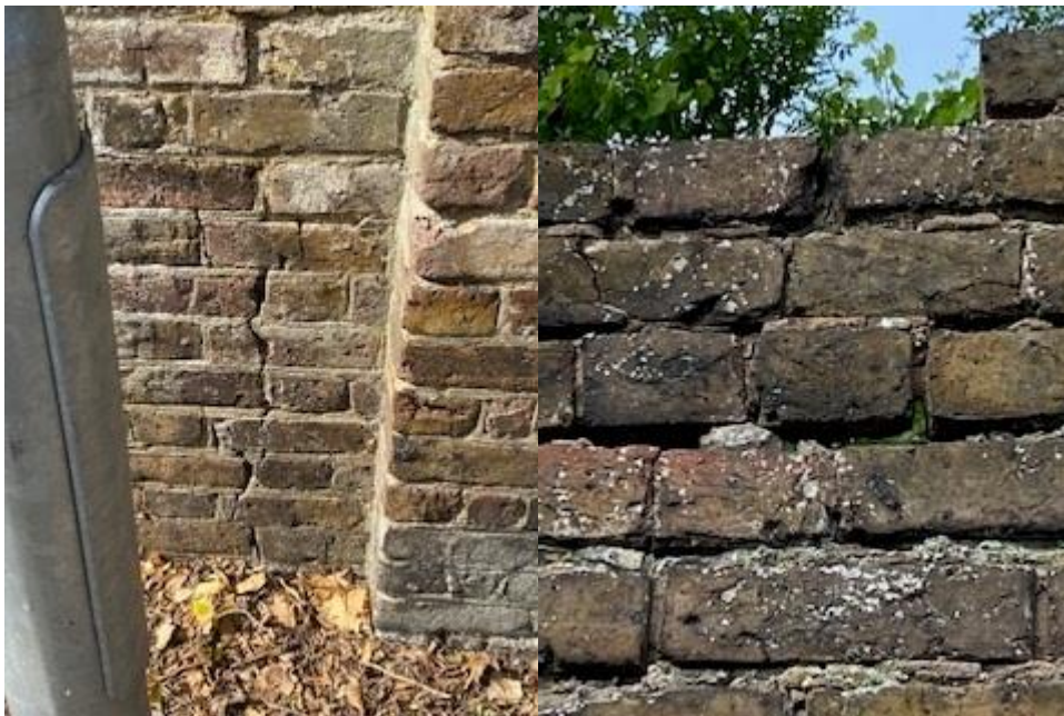
8. cracks in the wall and mortar is needed.
