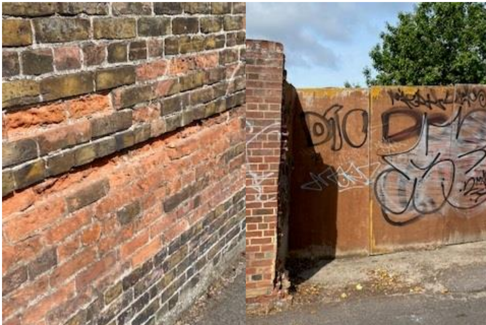
6. Replacement of bricks on the wall and bricks removed, wooden boards in place.
