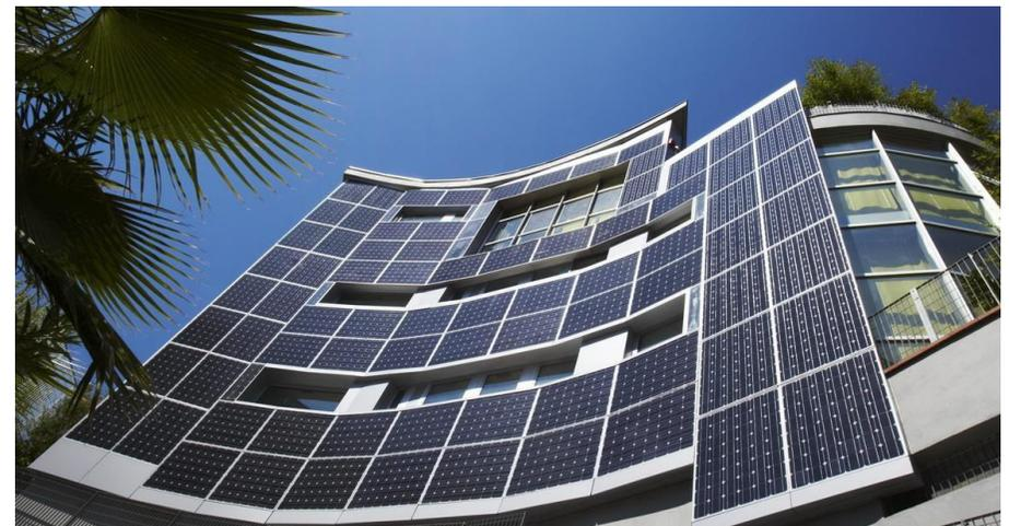
*South facing solar facades produce around 15% less energy than an East/West concertina array, but generate more electricity than an East/West array in winter months. For buildings with heat pumps, this can be a great match.*
