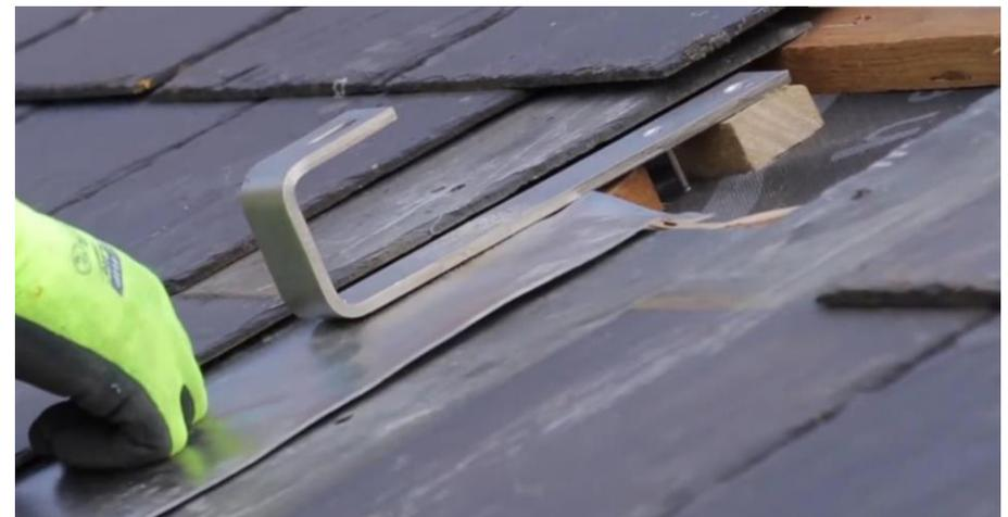
*Products and processes have been specifically developed to securely fit panels to existing roofs. Example shows a stainless steel roof hook being mounted to a slate roof.*
