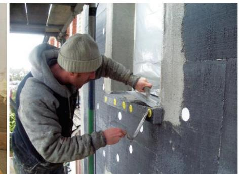
Photo of window install in Enerphit retrofit
