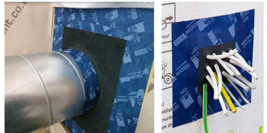
*Services entries present a risk to airtightness, however proprietary grommets are available to ensure airtightness can be achieved. The image on the left is of a ventilation duct as a reminder that airtight buildings must have a robust ventilation strategy.*
