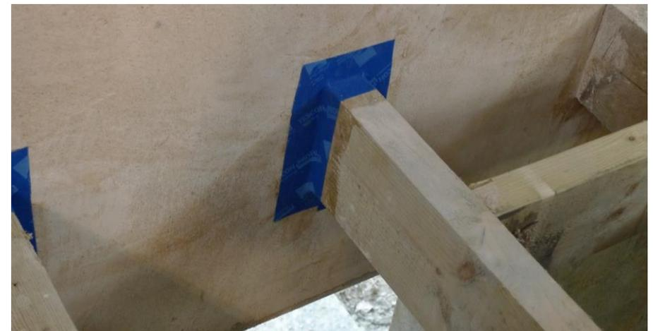
*Applying airtightness tape to joist ends is a common measure required to achieve good airtightness in existing buildings. Large gaps may need filling with mortar first, and remember to apply a suitable primer.*
