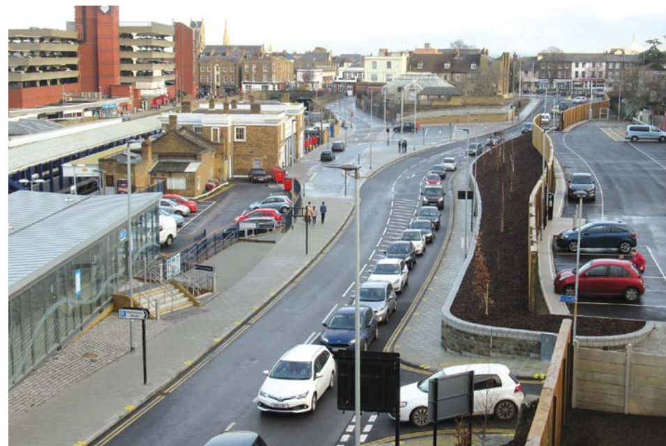
Rathmore Road completed improvements in Gravesend
