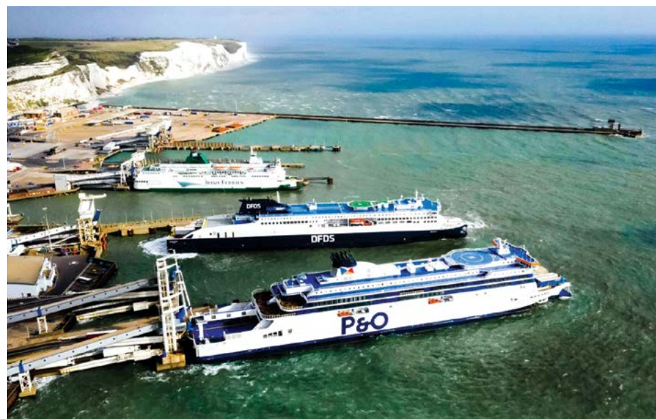
Port of Dover
