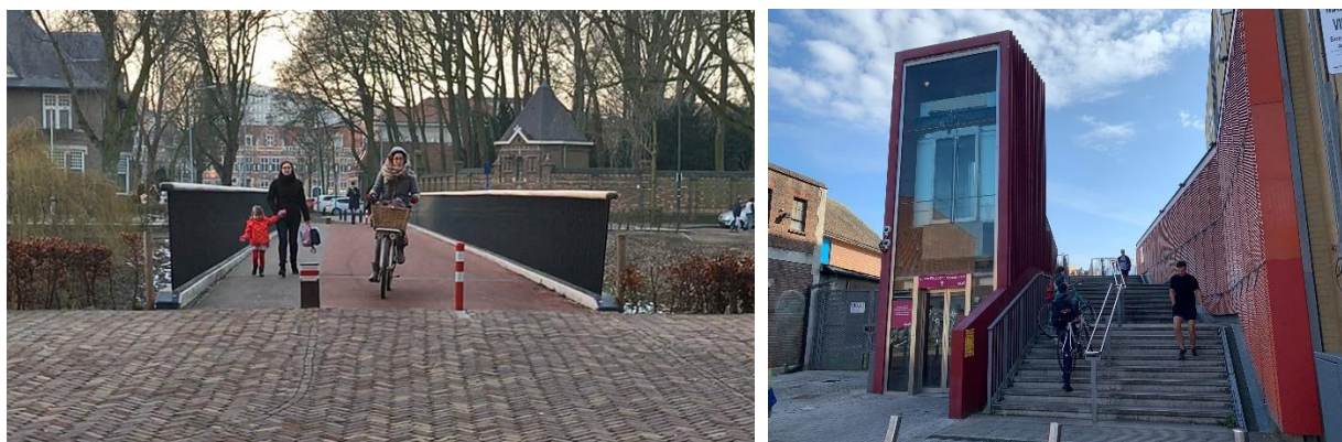
Figure 34: Example of a pedestrian + cycle bridge (Left – Mariabrug) and example of a new bridge incorporating access for steps, lift and ramps (Right – Wallis Road, Olympic Park)
