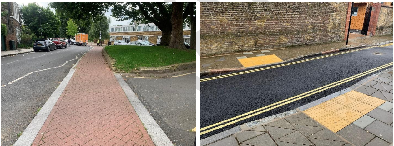
Figure 32: Continuous footway provision (Left – Claylands Road) and Dropped kerb with tactile paving (Right – Sans Walk)
