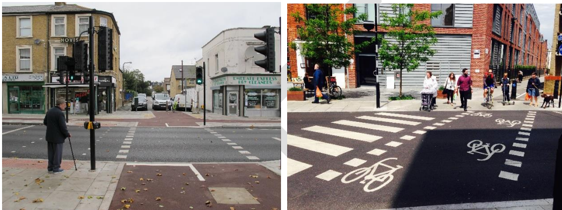
Figure 23: Controlled pedestrian & cycle crossing (Left - Lea Bridge Road), and parallel zebra crossing (Right – Richmond Road)
