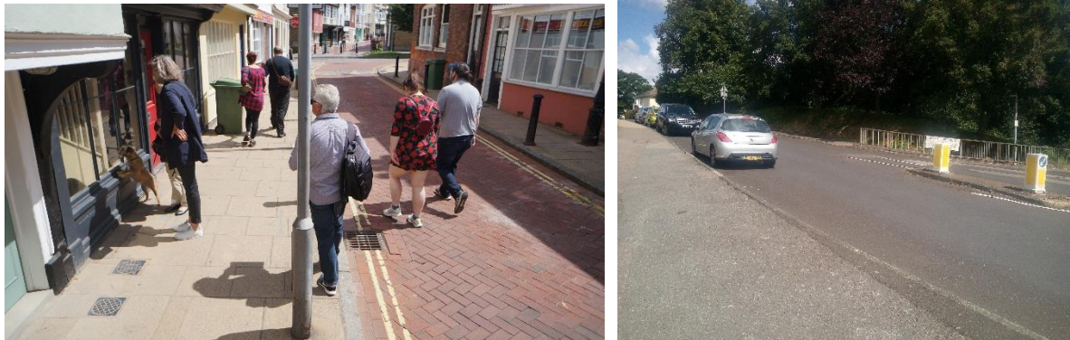
Figure 29: Narrow footway (West Street); Pedestrian crossing away from desire line (Bramblehill Road)
