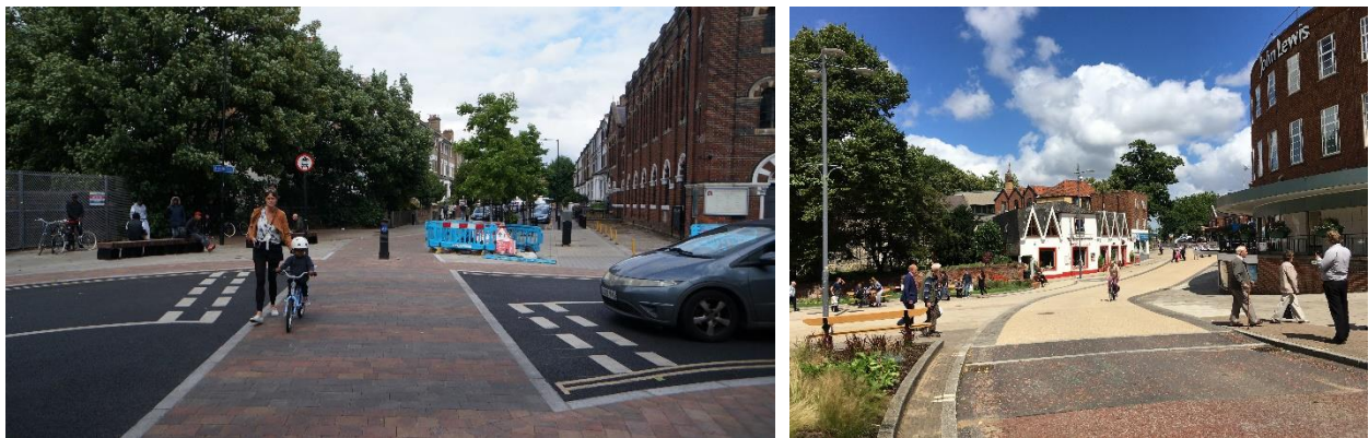
Figure 30: Implied crossing provides direct crossing on pedestrian desire line (Left- Downs Road), and example of a raised table crossing in Norwich (Left – Westlegate)
