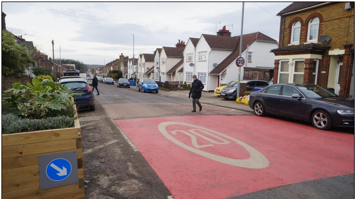
Figure 2-2: 20mph gateway feature
