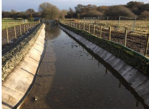
Over time the reed bed (into which the leachate flows) became blocked and required a significant upgrade to ensure enhanced environmental protection to the River Stour. The works will help ensure that any contaminants that are treated through the Plant, which have leached from the close by closed landfill site cause the absolute minimum disturbance to the close by and wider environment.
