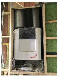
Image of Zehnder MVHR unit being retrofitted into an existing house (© Bowtie construction)
