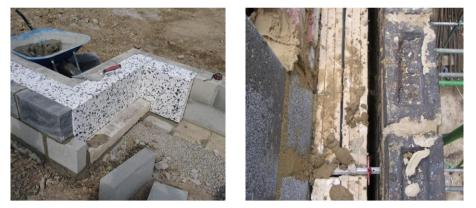
Left: an example of good Expanded Polystyrene insulation installation. Right: An example of poorly installed partial cavity installation, loosely fitting, and cement dropped atop and inside cavity.
