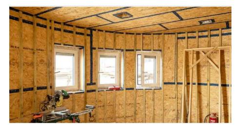
A good airtightness strategy forms the basis of an airtight building. This is an excellent example of taped OSB, with a dedicated service cavity on internal walls. The service cavity means most wires and pipes will not breach the airtight OSB layer.
