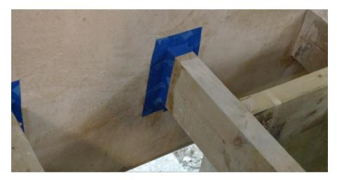
Applying airtightness tape to joist ends is a common measure required to achieve good airtightness in existing buildings. Large gaps may need filling with mortar first, and remember to apply a suitable primer.
