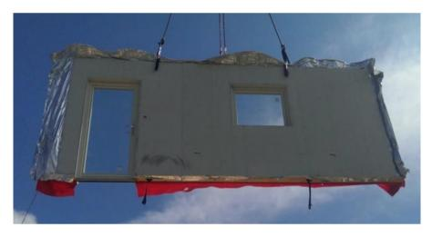
A closed-panel timber frame, manufactured off-site with insulation, window and door frame included (© Vision Development).
