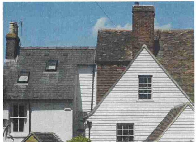
Adjacent steep slate and clay tile roofs; one with bell cast end
