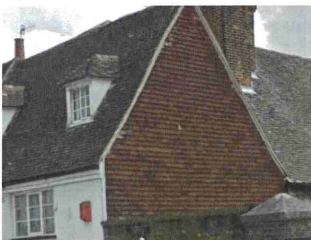
Peg tiles as wall cladding
