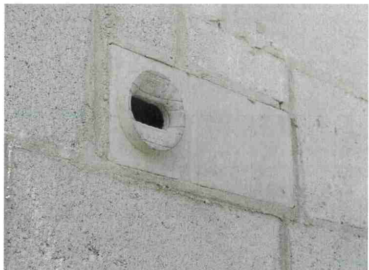
Integrated swift box, Nansleden (source: Duchy of Cornwall)
