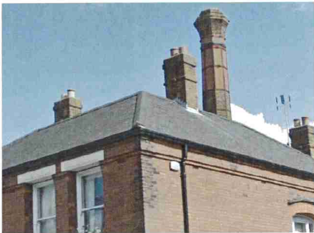
Slate roof with minimal eave
