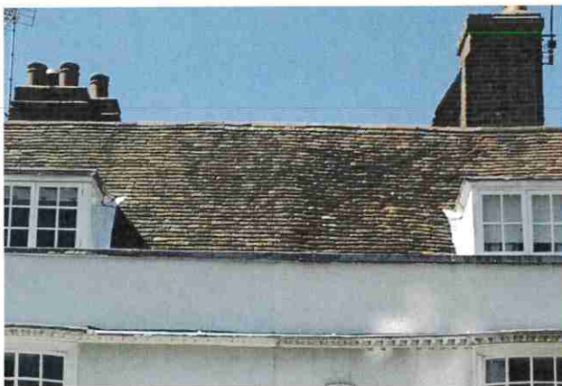
Clay tile roof with parapet
