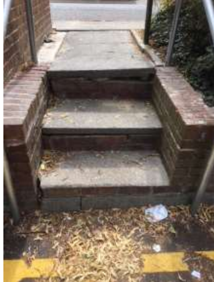
Thomas Road Car Park: Known trip hazard on steps. Gap under top steps, needs re-laying
